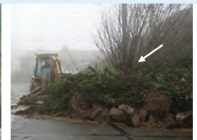
earth flow (unchanneled flow)
