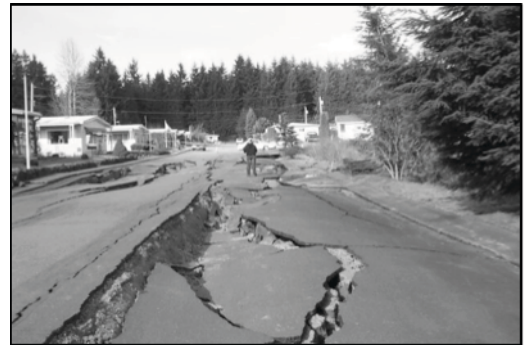
Image of damage from the 2001 Nisqually earthquake near Seattle
