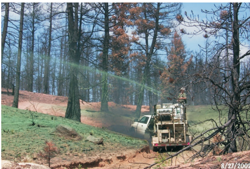
Figure 38 —Ground application of hydromulch aimed at reducing soil erosion.
